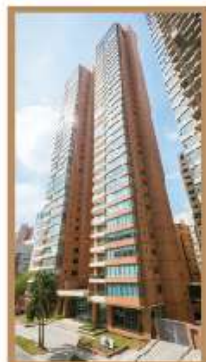
SOLARA TOWERS BARRANQUILLA
